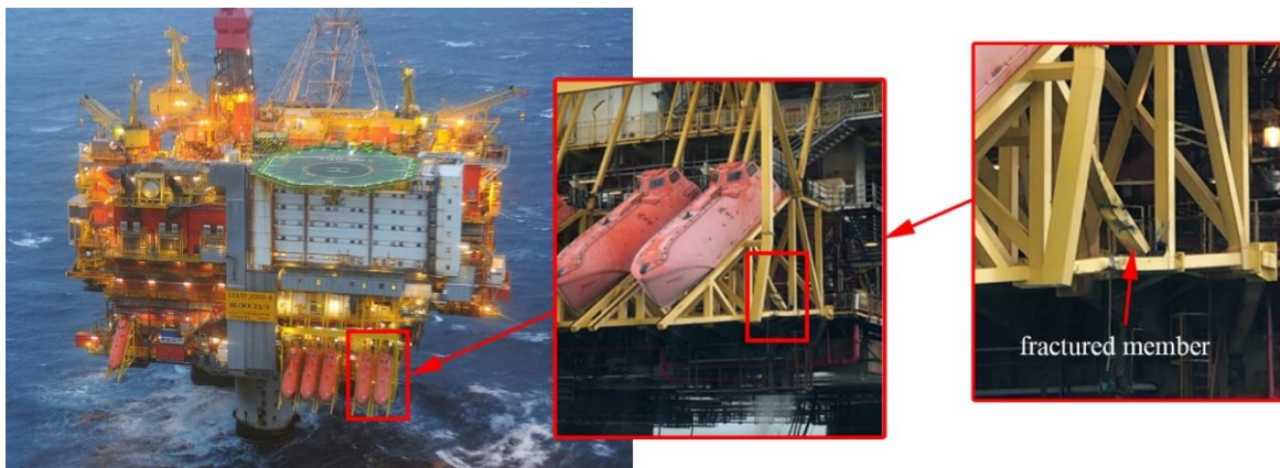
Figure 1.8. Sjøborg supply vessel collided with the Statfjord A platform and caused damage to the lifeboat structure in 2019 [59, 66].
